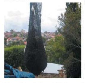
Left: Cleaning the SQID by lifting out the trash basket from the SQID.
