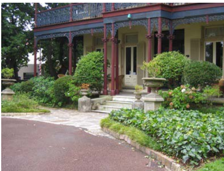
Verandah with sandstone step edging and cast iron columns and panels, 2007 (Source: OCP)
