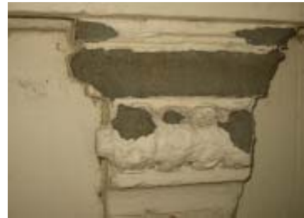
Deteriorated bracket underneath window sill, 2007 (Source: OCP)
