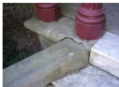
Cracks in verandah caused by sinking of front steps and parapet wall, 2007 (Source: OCP)
