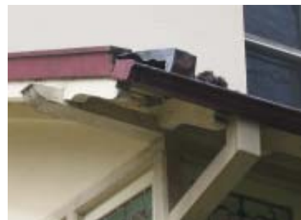
Skillion roof gutter sagging and full of leaves, 2007 (Source: OCP)
