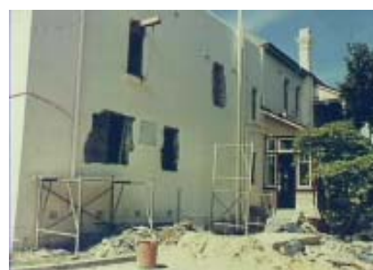
1986 Restoration work photograph showing the removal of the 6 louvered windows and reconstruction of 4 double hung windows to the west side of the rear wing of Boronia (Source: Clive Lucas Stapleton)
