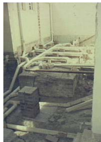
1986 Restoration work photograph which indicates that the floor of the rear wing of Boronia was raised up at the time it was occupied by Mosman Library (Source: Clive Lucas Stapleton)
