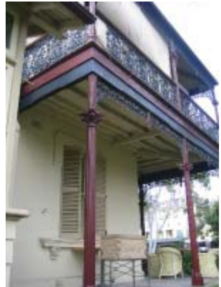
Cast iron columns and decorative cast iron balustrade, 2007 (Source: OCP)
