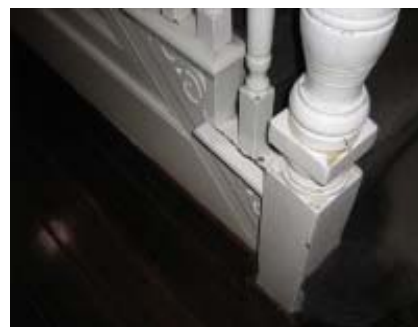
Cracks in treads of staircase, 2007 (Source: OCP)
