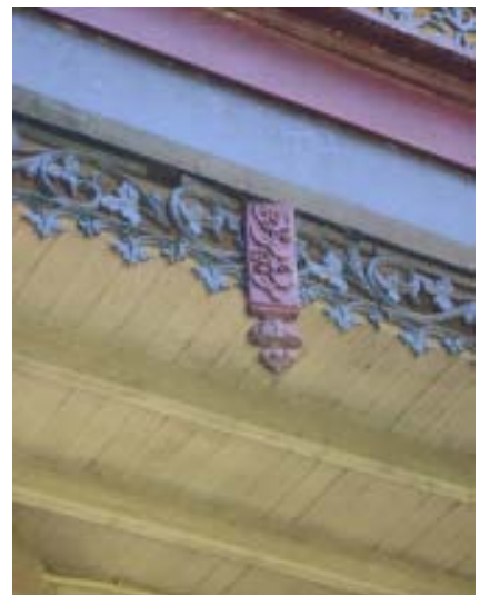
Part of cast iron valance showing panels and cast iron frieze drops, 2007 (Source: OCP)
