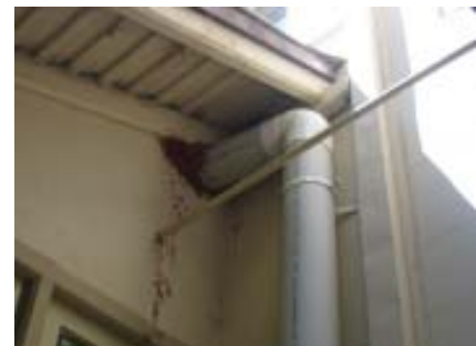
PVC pipe along glazed bay area with urethane sealant having leaked out of gaps, 2007 (Source: OCP)
