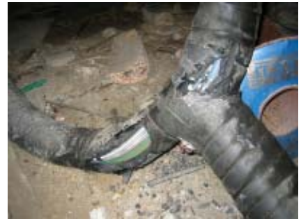
Sub-floor, damaged drink dispensing pipe, 2007 (Source: OCP)
