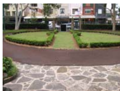
Pink-tinted bitumen used in circular carriage loop in sharp contrast to the bush stone crazy pattern paving. 2007 (Source: Gina Plate)
