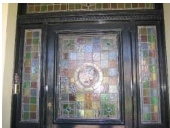
Entrance door with lead light panels, 2007 (Source: OCP)
