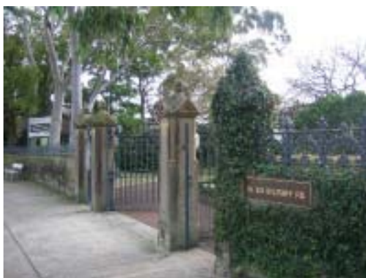
Stone boundary fence topped with decorative cast iron panels, 2007 (Source:Gina Plate)
