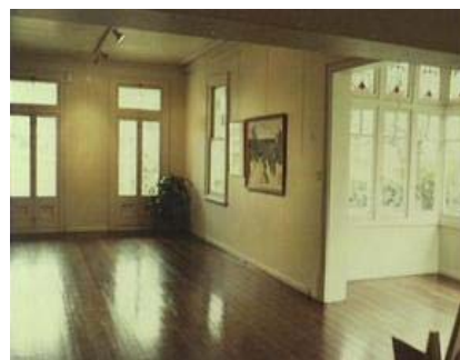
Glazed bay area with floorboards covering 1910 tiles, 1984 (Source: Mosman Library)
