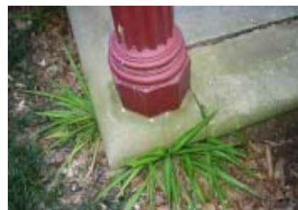
Subsidence of the south-east corner of verandah plinth, 2007 (Source: OCP)
