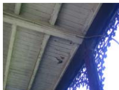
Metal roof of verandah has leaks and peeling paint, 2007 (Source:OCP)
