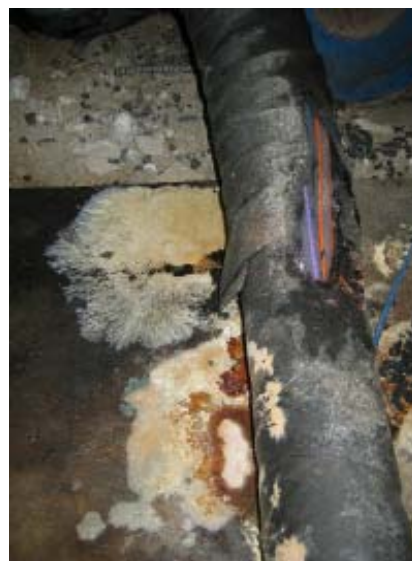
Eroded drink dispensing pipe, 2007 (Source: OCP)
