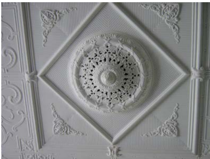
Original metal pressed ceiling, 2007 (Source: OCP)
