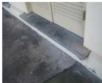
Delamination of slate thresholds of French doors, 2007 (Source: OCP)
