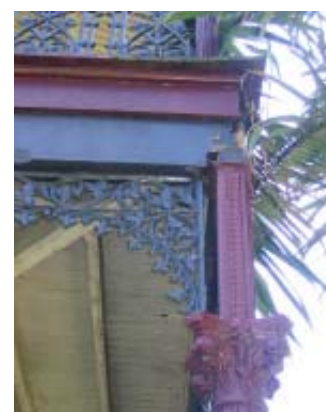
Severely damaged timber beam south-eastern verandah corner, 2007 (Source: OCP)
