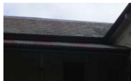
View of hipped roof showing missing tiles and tiles that need to be replaced, 2007 (Source: OCP)
