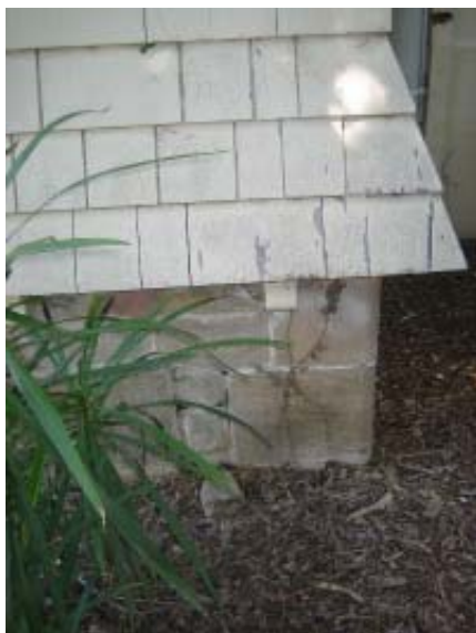
Deteriorated paint to wooden shingles on glazed bay area wall, 2007 (Source: OCP)
