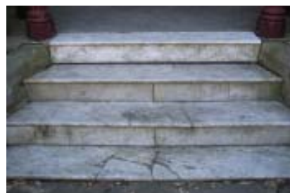
Cracked marble treads and risers of steps leading up to main entrance, 2007 (Source: OCP)
