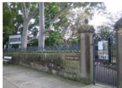
Front boundary wall with sandstone base topped with cast iron fence, 2007 (Source: OCP)
