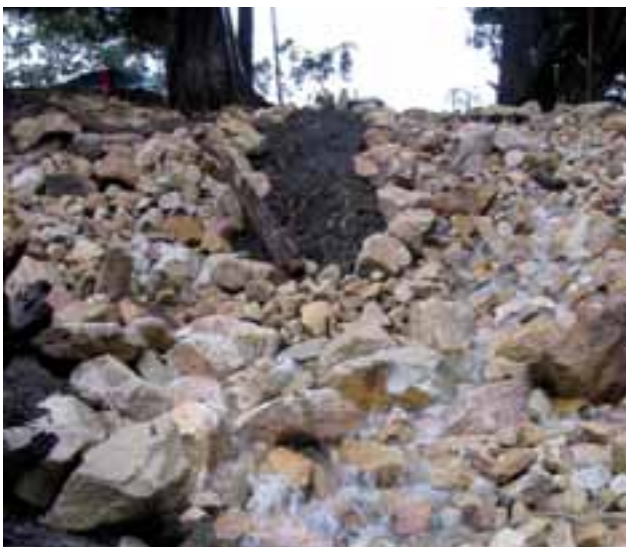
Creek armouring undertaken for the Red Crowned Toadlet project
