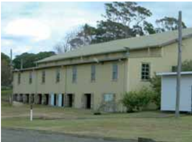
Council may implement a water reuse project at the Drill Hall Precinct, if leased from SHFT.
