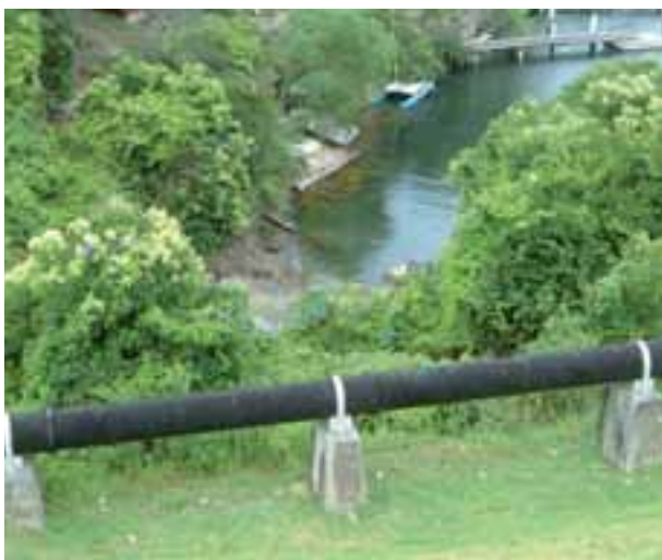
Above: Recently acquired land at Julian St before construction works to install a SQID began.
