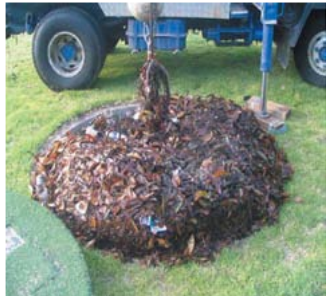
Above: Cleaning the Nettech device at Gordon Street, upstream of Lawry Plunkett Reserve.
