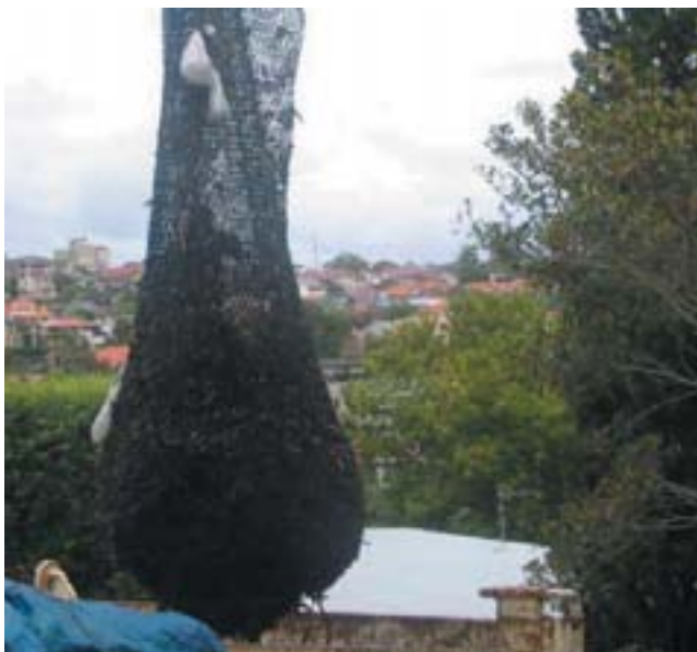
Above: Cleaning the Nettech device at Gordon Street, upstream of Lawry Plunkett Reserve.
