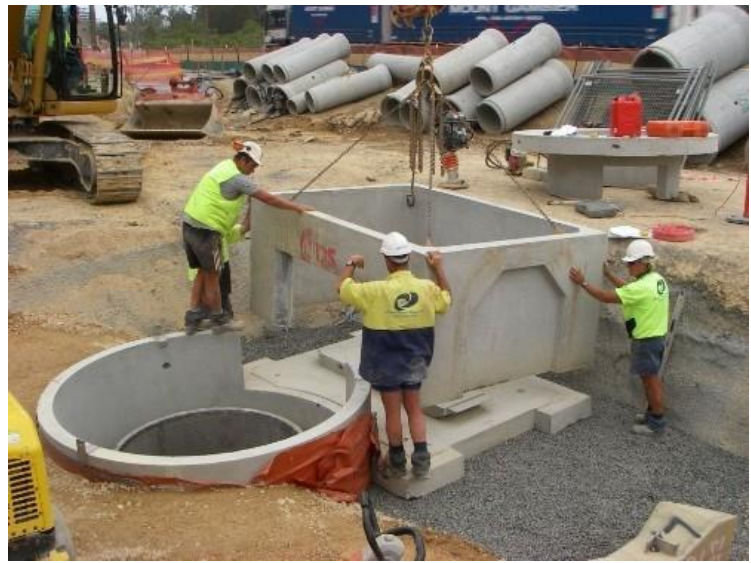
Pit with screen being installed
