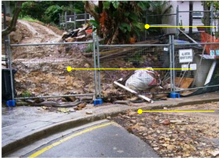
Inadequate erosion and sediment control measures
